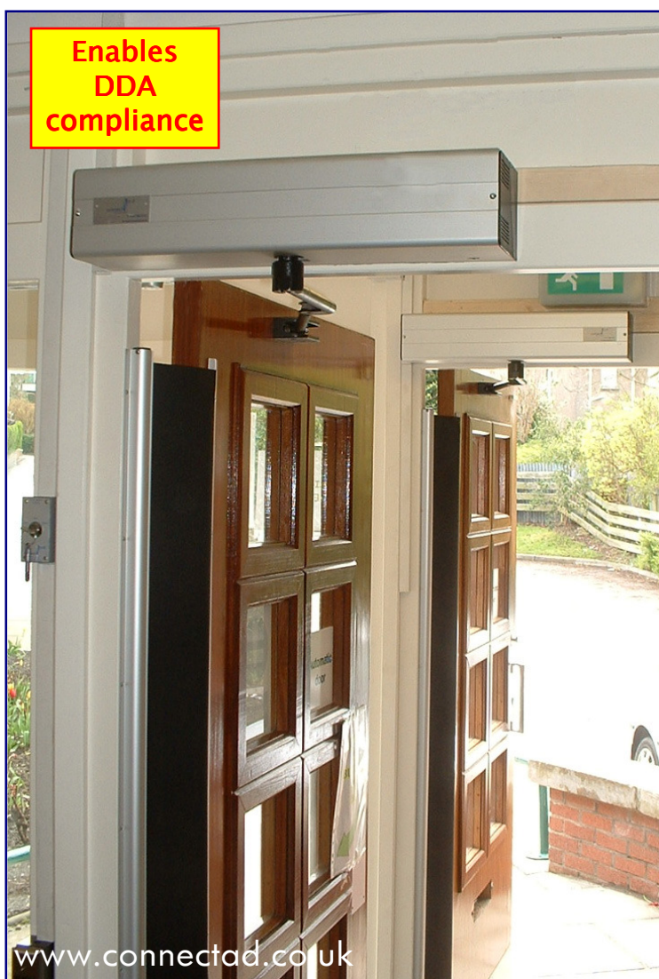
Retrofit installation by connect a.d. at a medical centre
