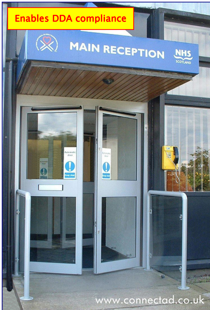
Manufactured and Installed by connect a.d. at a Healthcare Facility
